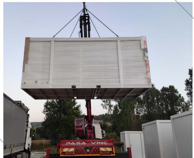
11 Cabin positioned with telehandler
