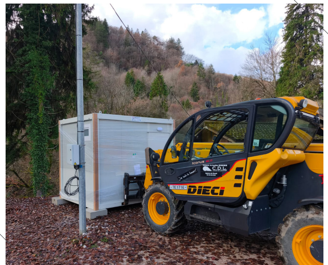
05 WC cabin positioned with telehandler
