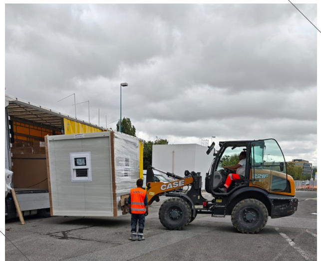
16 Forklift moving modular cabin
