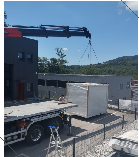
08 Crane unloading flat-pack unit
