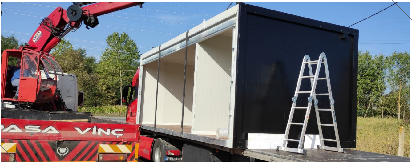
14 Crane positioning modular cabin
