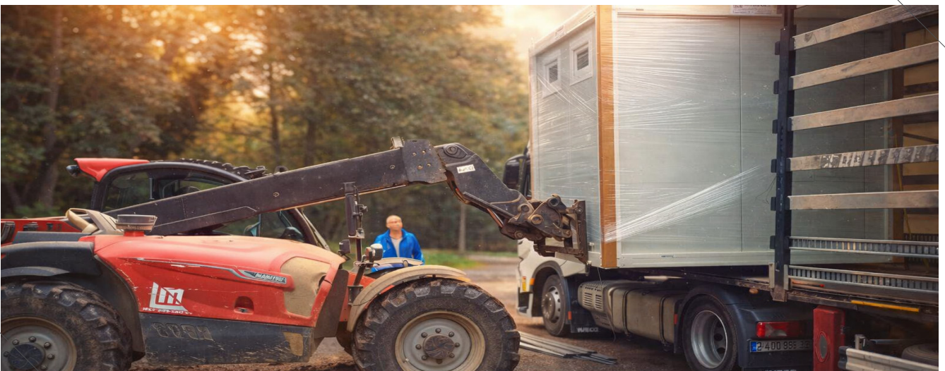
03 Module transfer from truck
